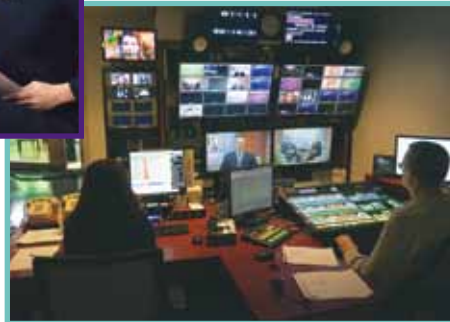
WBNG control room
